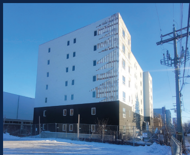
380 Young Street - 69 Residential units
